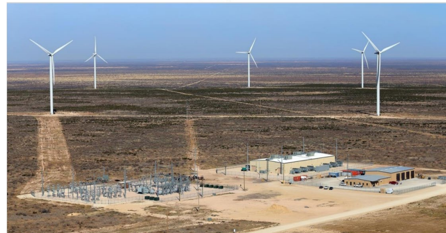
DOE Peer Review Notrees Energy Storage Project
