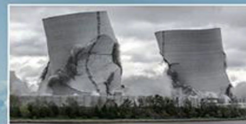
VIDEO: Watch the implosion of Brayton Point's two 500-ft. cooling towers (April 27, 2019)
