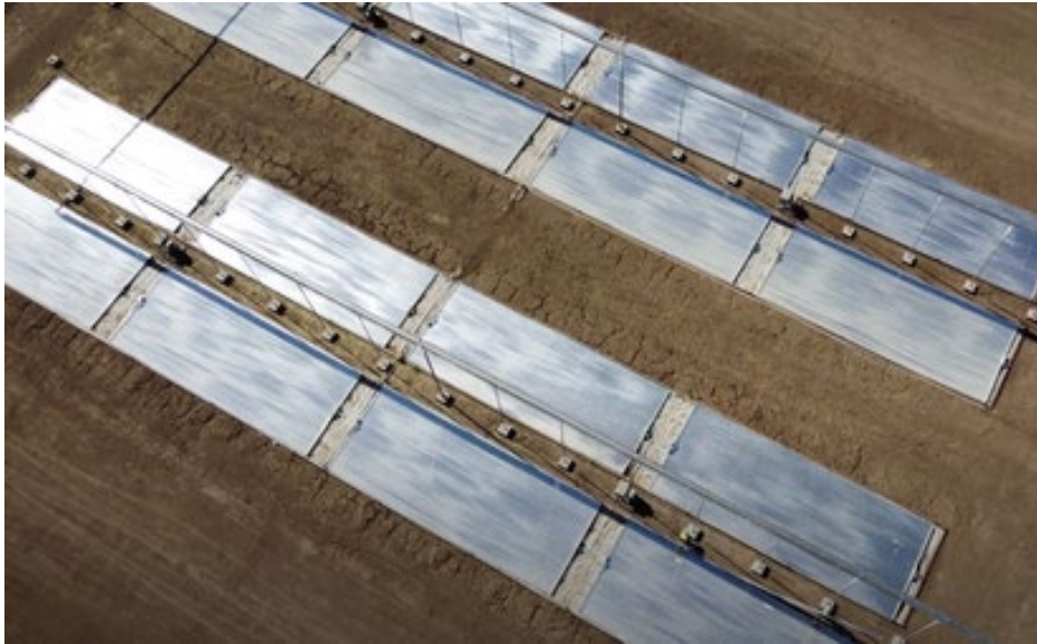
Tectonic Sun Alpha: First pilot plant in California to demonstrate application of concentrated solar paired with 6-month duration geothermal storage, turning existing oil wells into clean energy generators
